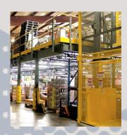
Mezzanine framing can be customized for a wide range of applications from small light-duty work platforms to large-span, heavy-duty industrial mezzanines.
