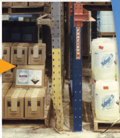
Roll-formed column on left, structural steel column on the right. The evidence of structural steel superiority is clear.
