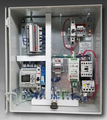
VRC Fault history is conveniently saved in the SmartControl™ PLC's memory while error messaging can be easily accessed on a digital panel inside the control cabinet for quick diagnosis by a qualified technician or an electrician.
