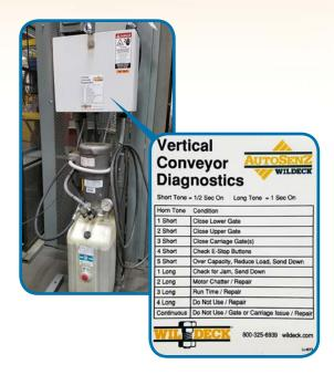
For the operator, SmartControl™ placards are available at each lift station to describe ten potential fault conditions that are annunciated via the system's audible alarm.
